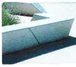
PRECAST CONCRETE WALL / SEAT
